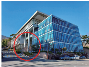
Main Entrance Foreground
