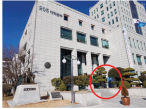
Main Admin. Bldg. Front Left Entrance
